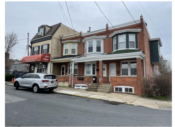
Single Family Row Houses and Commercial
