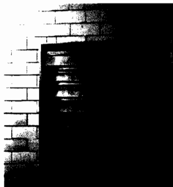
Two Gravity Louvers Located in Duct Room To Be Cleaned Annually
