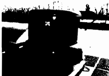
Cook Ventilator EF-2 Model No. 330ACE 330C8B S/N: 076SE49822-01/0000702 1.5 Hp; 8520 CFM; 460 V; 3 Phase Jan-13 Belt: AX-39
