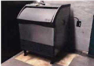
Ice Machine - Porter Operator's Area Scotsman Brand Model CU1526SA-1A Serial No. 17011320014000 Refrigerant Charge: R404A 115 V; Single phase; 7.7 Amps
