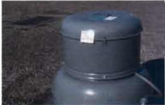
Cook Ventilation Unit EF-7 Model No. 120ACE 120C3B S/N: 076SE 49822-01/000-4401 0.25 Hp; 650 CFM; 115 V; 1 Phase Jan-13
