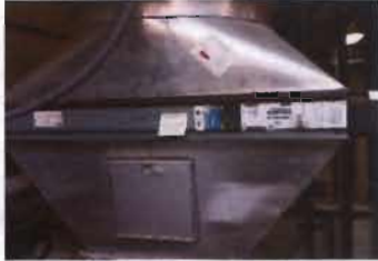
Duct Heat Exchanger - 24" x 42" Steam Trane Coil Type NS Sigma Flo Serial No. H12E04661 Order No. D2T823A B/L A Air from a roof top unit Location: Near rear entrance
