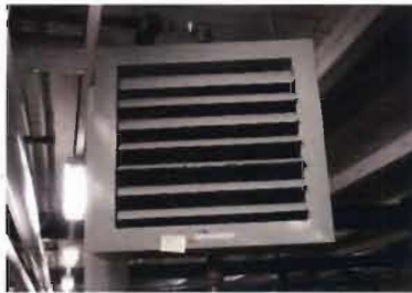
Hydronic Unit Heater Modine Model No. HSB193SB01SA (Year: 2018) Serial No. 43104517-1285 1/3 Hp; 115 V; 4.2 Amp Location: No. 4 Sed Basin - north
