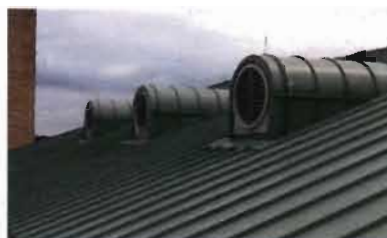
Exhaust Fans - Roof Top Pump Station Quantity: 5
