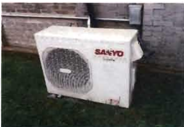
Sanyo Split Unit Model No. CH0971 Serial No. 0105212 85221344550000 115 V, Single Phase Plant Supv Office
