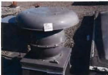
Cook Ventilation IF-3 Model 120CVR S 120CVR SVP S/N: 076SE49822-00/0003801 0.25 Hp; 650 CFM; 115 V; 1 Phase Jan-13 Louvers to be cleaned annually
