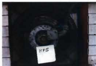
Exhaust Fan Penn Ventilator Model P10V B2W Location: Bathroom in Pump Station Direct Drive
