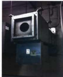
Exhaust Fan - EF-2 Location: Pump Room Greenheck Model No. BSQ-70-4 Serial No: 06H26878 Belt: 3L-360
