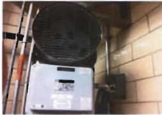
Chromolox Electric Unit Heater Model: HD3-500 208 V; 5 KW; 3 phase; 0.6 Amp
