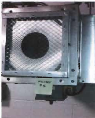
Exhaust Fan EF-2 Greenheck Model BSQ-70-4 12" Centrifugal Inline Fan Serial No. 06H26876 Belt: 3L-360R
