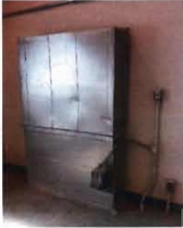
Damper No. 2 and 3 Motorized Wall Unit Ducted to Basement Location: Pump Room
