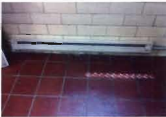
Electric Baseboard Heaters Quantity: 2 110 V; 15 Amp
