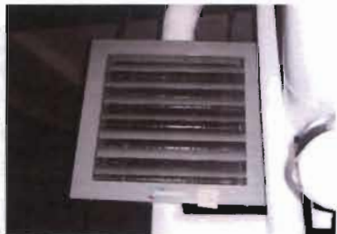
Hydronic Unit Heater Modine Model No. HSB193SB01SA (Year: 2018) Serial No. 43104517-1284 1/3 Hp; 115 V; 4.2 Amp Near Sed Basin No 7 South Side
