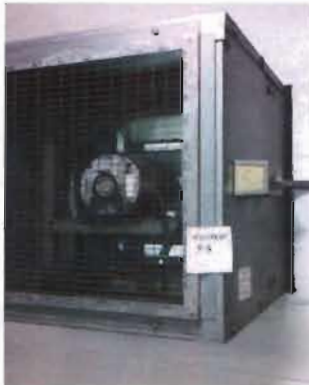
Exhaust Fan EF-1 Greenheck Model SE2-16-417-A3 16" Direct Drive Serial No. 06H26234 Direct Drive
