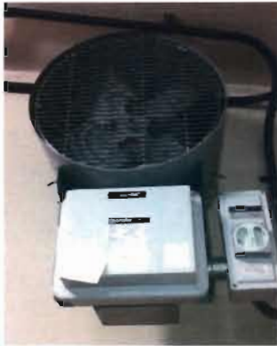
Electric Unit Heater - EUH-1 Chromolox Model No. HD3D-1000PST 004-305709-089 480 V; 10 KW; 3 Phase Location: Hypo Room
