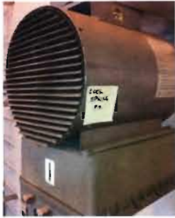
Electric Unit Heater - EUH-1 Marley Electric Heater Model No. W75041A MFG Code - L94 7.5 KW; 240 V; Single Phase Location: Pump Station
