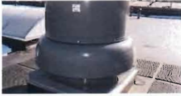
Model No. 330ACE 330C8B S/N: 076SE49822-01/0000702 1.5 Hp; 8520 CFM; 460 V; 3 Phase Jan-13 Belt: AX-39
