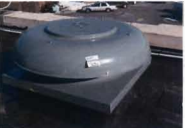
Cook Ventilator IH-2 Model No. 240PR 24PR S/N: 076SE49822-01/0006902 2650 CFM Jan-13
