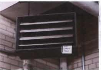
Loading Dock, Near Elevator Trane Steam Unit Heater Model No UHSA-038S-8C-AAC S/N: D91H08890
