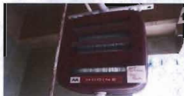
Steam Unit Heater Modine Model HS47S01 Serial No. SP011996 Location: Tool Room
