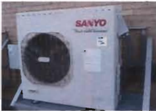
Split Unit on Roof Sanyo Flexi Multi Inverter Model CMH 3172 S/N: 0012193 85221344585002 230 V; single phase Date: July 2009
