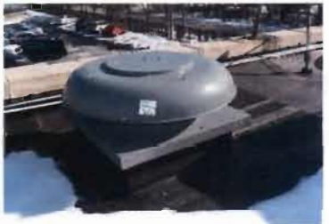
Cook Ventilator IH-1 Model No. 240PR 24PR S/N: 076SE49822-01/0006901 2650 CFM Jan-13
