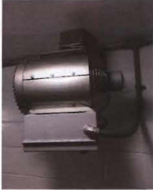
TPI Corporation Model P3P5507T Quantity: 1 480 V; 7.5 KW; 3 Phase, Wall Mount Thermostat
