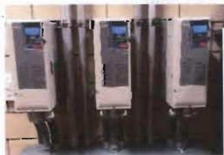
Yaskawa VFD Controllers Z1000 Model VFD's control Louvers 200 V 10.6 Amp
