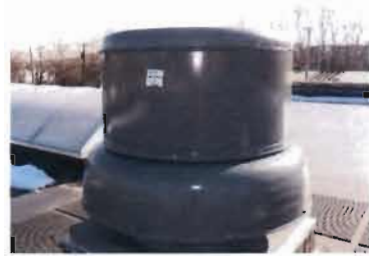
Cook Ventilator EF-1 Model No. 330ACE 330C8B S/N: 076SE49822-01/0000701 1.5 Hp; 8520 CFM; 460 V; 3 Phase Jan-13 Belt: AX-39
