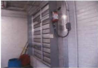
Louver Vent 2 Electric Actuators 60" x 72" Honeywell MS811A1206 Serial No. 0941GZU2026 Serial No. 0947GZU3082 Location: Sed Basin 8-10
