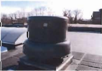
Cook Ventilator EF-3 Model No. 330ACE 330C8B S/N: 076SE49822-01/0000703 1.5 Hp; 8520 CFM; 460 V; 3 Phase Jan-13 Belt: AX-39 Louvers to be cleaned annually
