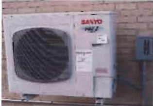
Split Unit on Roof Sanyo R410A Model C3672R S/N: 0020911 230 V; 13.8 Amp; single phase
