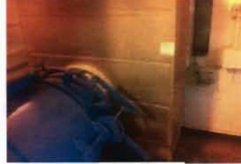
Exhaust Fan - EF-2 Twin City Fan and Blower Size 182; Type: BCV ARR. 10; Serial No. 7818612 With Actuated Damper Belt: 4L-330
