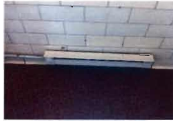
Electric Baseboard Heaters Quantity: 2 110 V; 15 Amp
