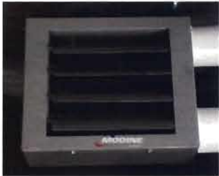
Serial No. 39104018-5093 1st Floor of Gate House
