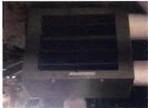
Two Hydronic Unit Heaters: Modine Model HC 24SB01SA 1/25 Hp; 115 Volt; 1.3 Amp
