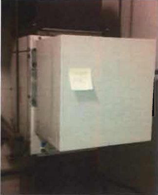
Exhaust Fan EF-1 Location: Hypo Room Greenheck Model No. BSQ-70-LMD Serial No. 10824850070 Belt: A-36
