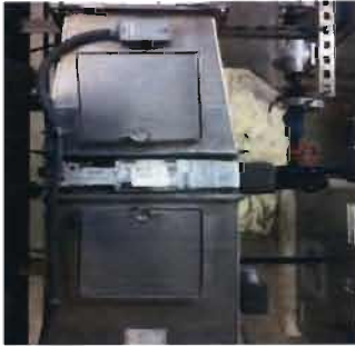
Duct Heater Heat Exchanger Trane Coil Type: NS Sigma Flo Serial No. H12E04662 Order No. D2T823A Serv. Model No. DNSB12016GOAA064AADA00B0000 Coil Serial No. 122012060B Location: Membrane floor, above air compressors - (Photograph view from above)
