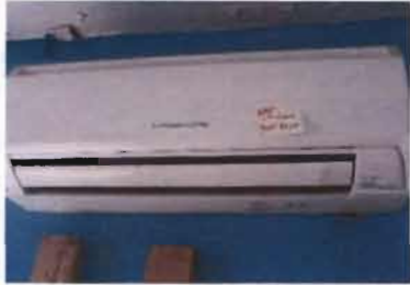
Mitsubishi Electric Heat Pump, Split System Model No MSZ-A17NA Serial No. 6003457-T 208 V; 1 Phase Location: 2nd Floor Shop Area
