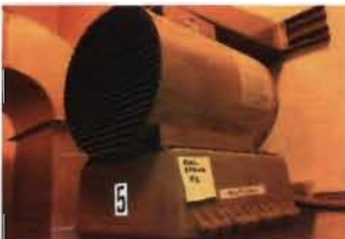
Electric Unit Heater - EUH-5 Marley Electric Heater Model No. W50041A Corrosion Resistant/Washdown MFG Code - L94 5 KW; 240 V; Single Phase Location: Pump Station
