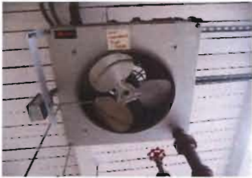
Steam Unit Heater Trane Model UHPB0801TAA4000004B Serial No. F12E32493 1200 CFM; 80,600 BTU/Hr Output 115 V; 1 Phase; 2.1 Amp Location: Membrane Feed Pump Room
