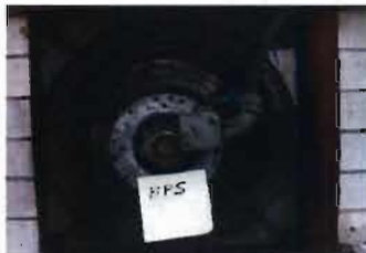
Exhaust Fan Penn Ventilator Model P10V B2W Location: Bathroom in Pump Station Direct Drive
