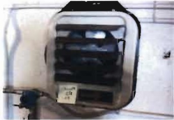
Marley Q-Mark Electric Unit Heater Model No MUH 0521 - 3700 Watts 21 Amps; 208/240 V; - Heater .25 Amp; 208/240 V - Motor
