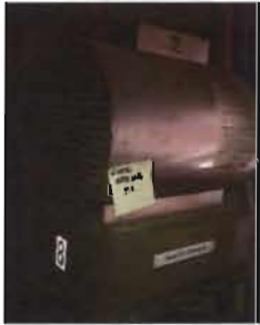
Electric Unit Heater - EUH-8 Marley Electric Heater Model No. W50041A Corrosion Resistent/Washdown MFG Code - L94 5 KW; 240 V; Single Phase Location: Pump Station
