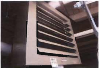
Hydronic Unit Heater Modine Model No. HSB193SB01SA (Year: 2018) Serial No. 43104617-1192 1/3 Hp; 115 V; 4.2 Amp Location: No. 10 Sed Basin - north
