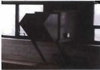
Odd Side Filter Area Belt Driven Fan 3' X 3' Wall Unit to Outside Extraction Air Belt: 4L-290R
