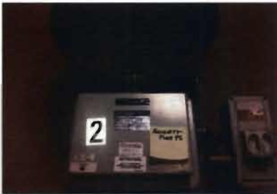
Electric Unit Heater - EUH-2 Chromolox Model No. HD3D-2000 004-305496-022 480 v; 20 KW; 3 phase Location: Pump Room
