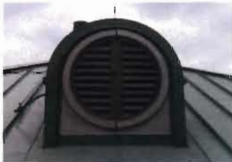
Exhaust Fans - Roof Top Pump Station Quantity: 5
