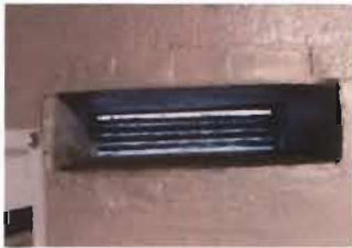
Fixed Slot Louver located in Chlorine Room. To be cleaned annually
