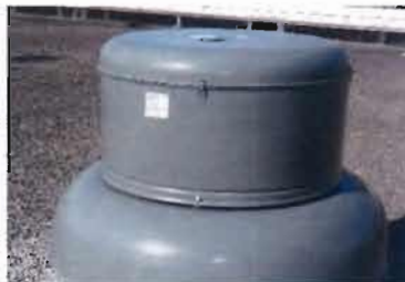
Cook Ventilator EF-5 Model No. 245ACE 245C6B S/N: 076SE49822-01/00020001 0.75 Hp; 5100 CFM; 460 V; 3 Phase Jan-13
