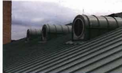
Exhaust Fans - Roof Top Pump Station Quantity: 5
