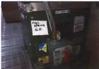
Exhaust Fan - EF-4 ILG Model No. 5508.SQDA08E16 Serial No. 081007M287820 Location: Cool Spring Gate House Direct Drive
