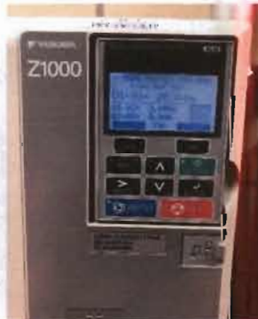
Yaskawa VFD Controllers Z1000 Model VFD's control Louvers 200 V 10.6 Amp
