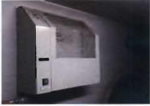
Chromalox Electric Unit Heater Cat No. HCH-051M 277 V; 1 Phase; 500 Watts EF-6 Valve Nook - Lower Level
