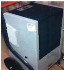
Portable Dehumidifier Dayton Model 2YV13 500 Watts July, 2012 Location: Basement
