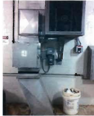
Exhaust Fan EF-4 Greenheck Model No. BSQ-120-5 Serial No. 06H26870 Location: Pump Room Belt: 4L-430 Includes Intake Louvers
