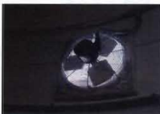
Lime Silo - Upper Dayton Fan Model 2C713B 1550 RPM; 1/20 Hp; 115 V; 1.8 Amp
