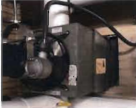
Carbon Room Modine Model HSB 33SB06SA 1/6 HP; 115 V; 2.1 Amp S/N: 18101819-5024
