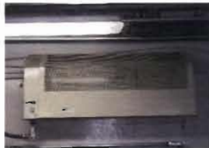
Chromalox Electric Unit Heater Cat No. HCH-501M 277 V; 1 Phase; 5000 Watts EF-8 - Lower Level Pump Area
