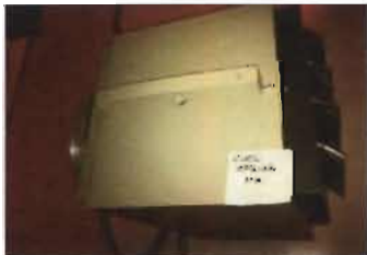
Electric Unit Heater - EUH-9 TPI Corporation Model No. H1HUH05003 240 V; 5.0 KW; Singl Phase Location: Pump Station, near Overhead Door
