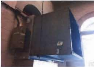
Exhaust Fan - EF-3 American Cool Air Model CBL/NBF 24SPUN Serial No. 062907M236240 Location: Cool Spring Gate House Belt: 4L-470
