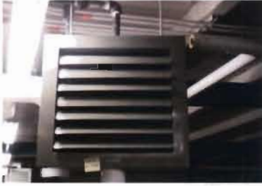
Hydronic Unit Heater Modine Model No. HSB193SB01SA (Year: 2018) Serial No. 43104517-1191 1/3 Hp; 115 V; 4.2 Amp Location: No. 8 Sed Basin - north
