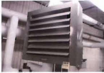
Hydronic Unit Heater Modine Model No. HSB193SB01SA (Year: 2018) Serial No. 43104417-2303 1/3 Hp; 115 V; 4.2 Amp Near Sed Basin No 1 South Side
