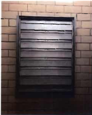
Two Gravity Louvers Located in Duct Room To Be Cleaned Annually
