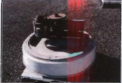
Westinghouse Fan Matches to Meter Shop 3/4 Hp; 115/230 V; 13/6.5 A S/N: 312P446 (Rarely Used) Belt: 4L-320
