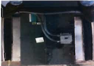
Duct Ventilator Loren Cook Model 150SON 10D Serial No 076SE49822-01/0005601 0.33 Hp; 800 CFM; 1075 RPM; 115 V; Single Phase
