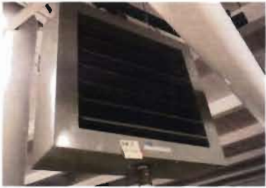
Hydronic Unit Heater Modine Model No. HSB193SB01SA (Year: 2018) Serial No. 43104517-1283 1/3 Hp; 115 V; 4.2 Amp Location: No. 2 Sed Basin - north
