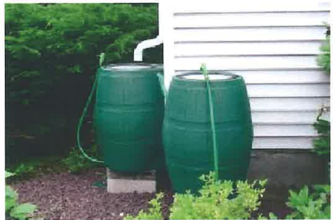
Example of rain barrels, similar to these offered for free by the Philadelphia Water Department's Rain Check Program
