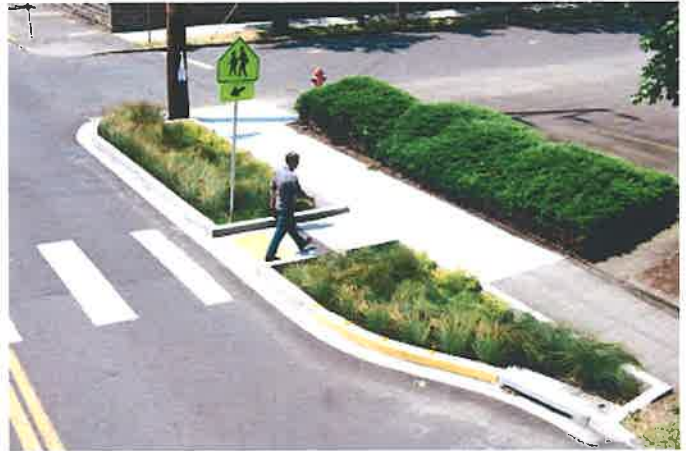
Example of a stormwater bumpout, one of the green infrastructure tools recommended in Philadelphia's Green Streets Design Manual
