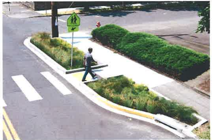
Example of a stormwater bumpout, one of the green infrastructure tools recommended in Philadelphia's Green Streets Design Manual
